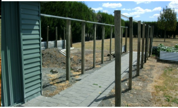
CURRENT : Walkway area with pavers now in place
