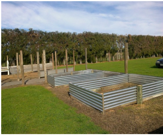
BEFORE : Area showing erected garden plots
